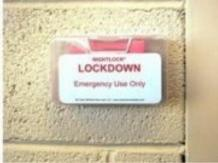
The Night Lock Locking Handles can be conveniently stored in a secure location within the classroom or office. A Wall Box is provided with each unit, and can be positioned anywhere in the room for quick access to the handle in case of an emergency lockdown event. The handle is red for quick and easy visibility. Most schools prefer positioning of the wall box near the door or at the teacher's desk as seen in the photographs above.
